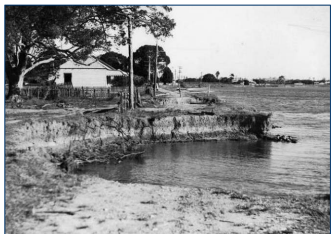
Erosion in Palmers Channel in 1946
