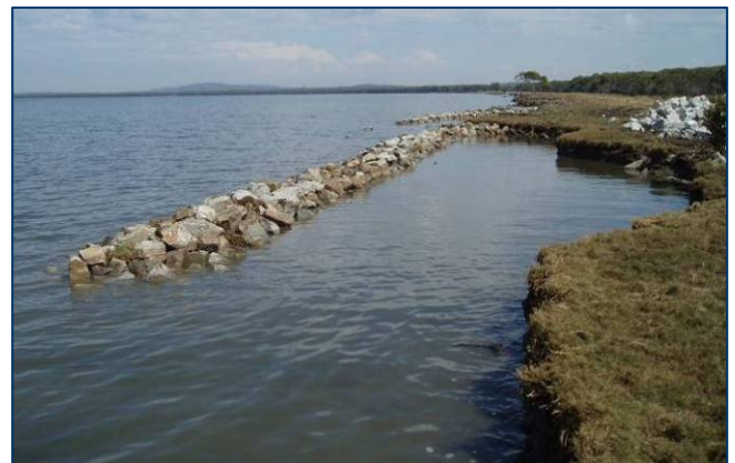
Intermediate treatment: Rock used to provide fish habitat and bank stability in Wooloweyah Lagoon
