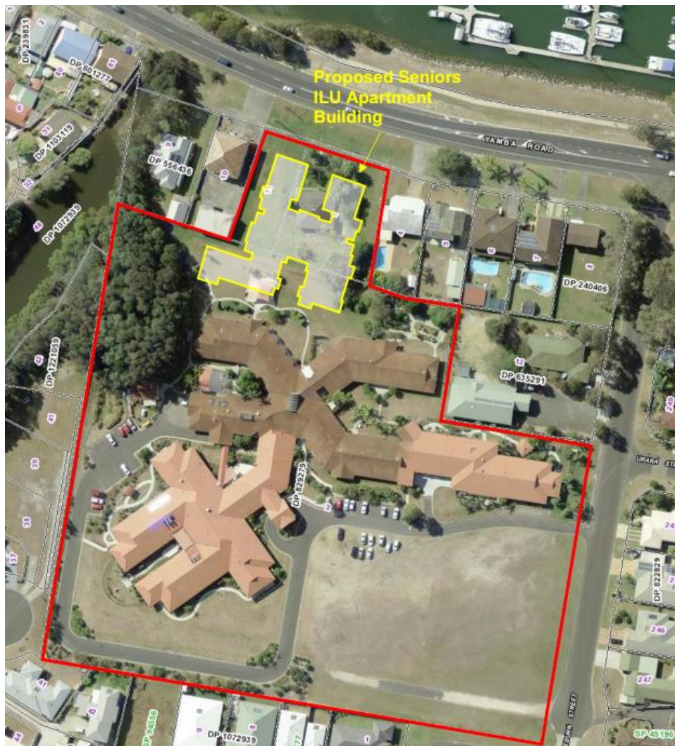
Figure 2: Aerial view of Uniting site
