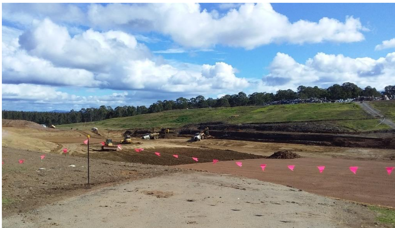
Figure 1 – Installation of clay liner
