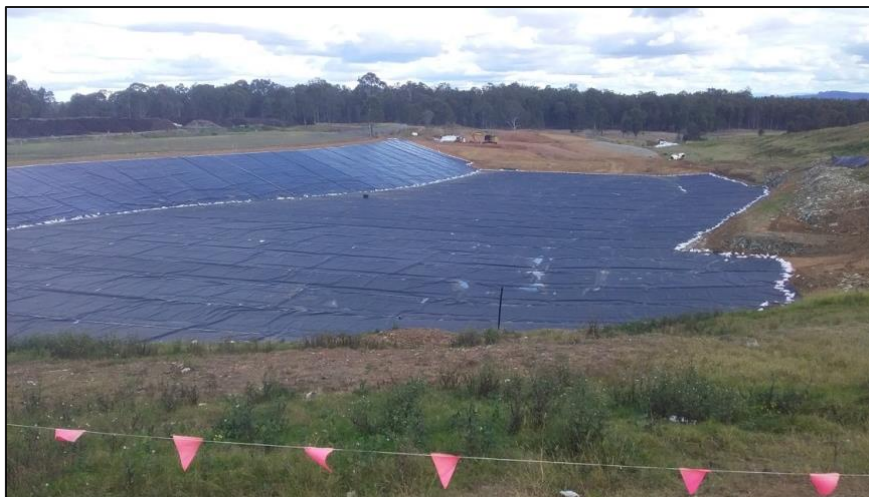
Image 2 – Installation of 2 mm HDPE Liner
