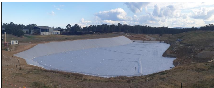
Image 4 – Installation of separation geotextile over leachate rock
