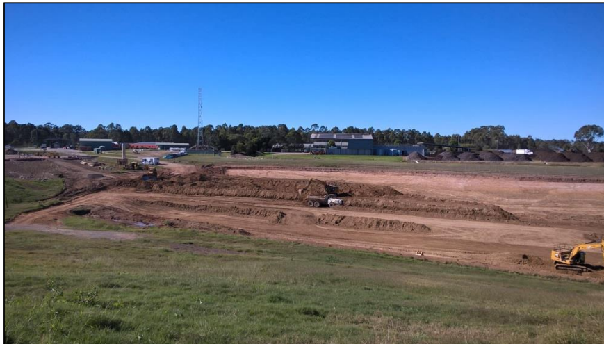
Image 1 – Bulk excavation of 180,000 tonnes clay
