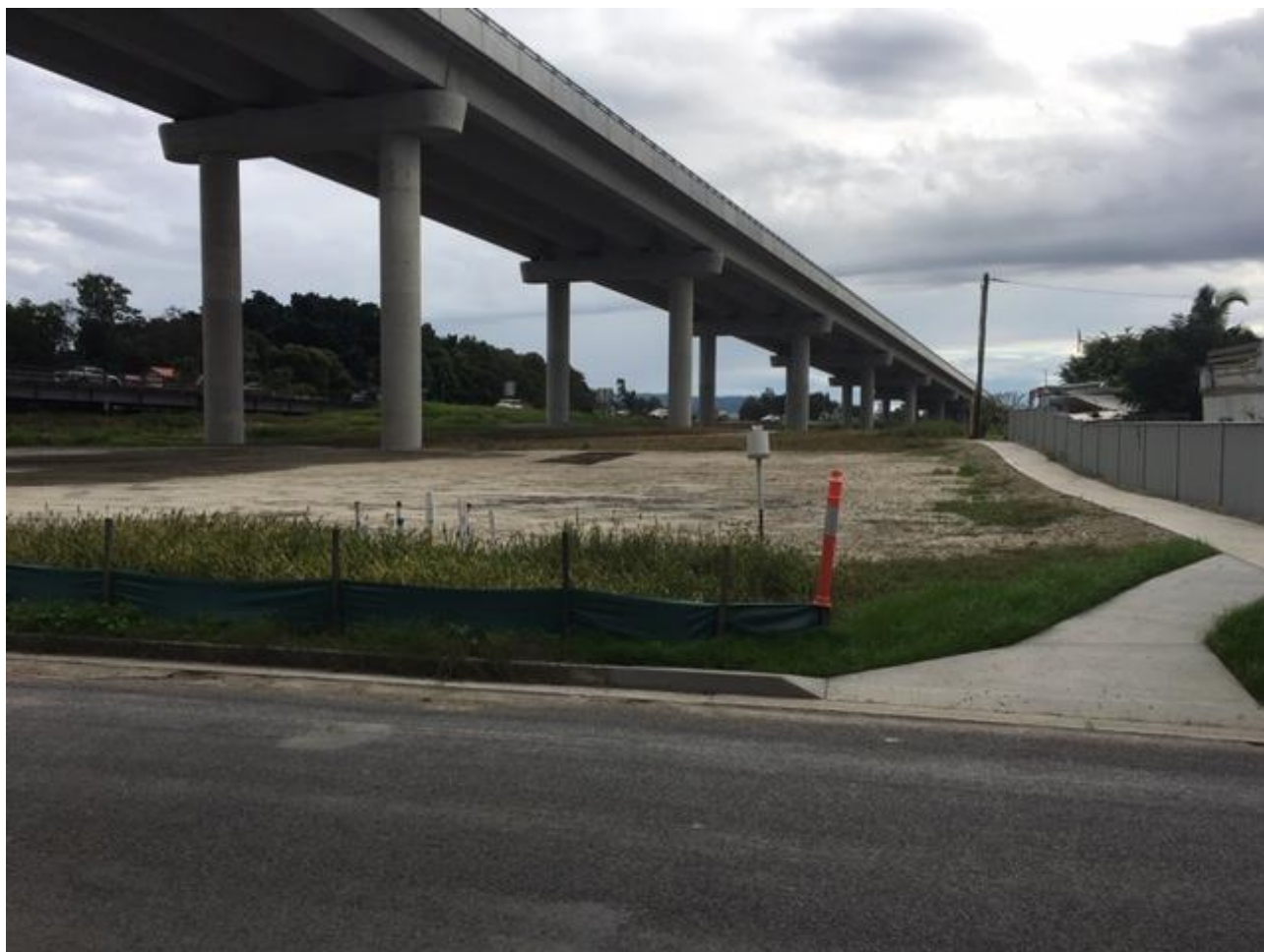
Figure 1 - Harwood Bridge Area
