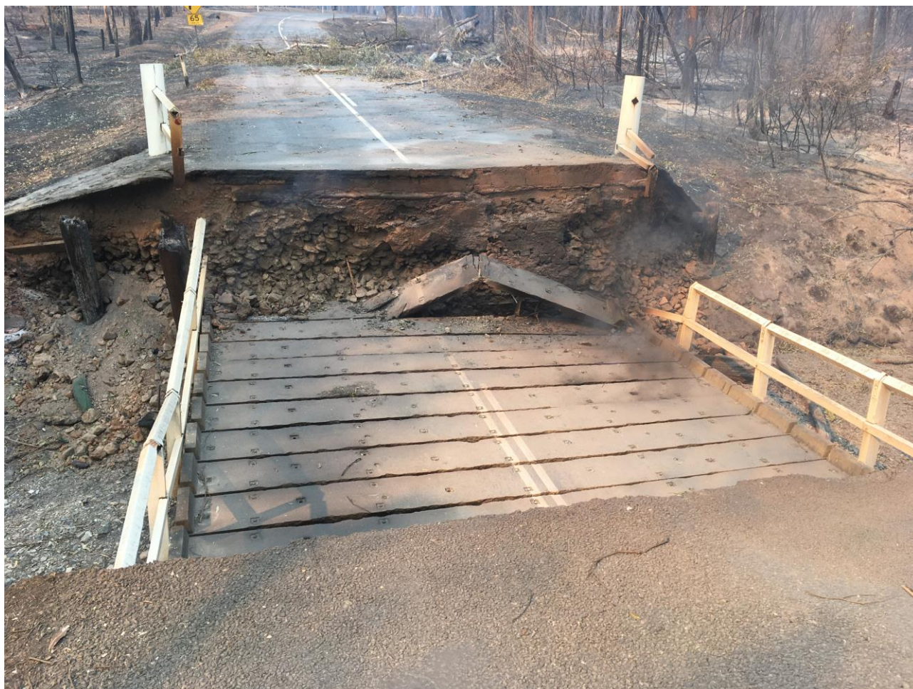
Figure 1 – Hortons Creek Bridge
