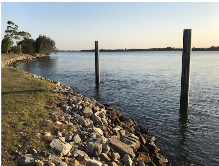
Figure 1 shows location of the existing piles looking south, the pile on the left is to be retained and made the new northern pile. (photograph by applicant)
