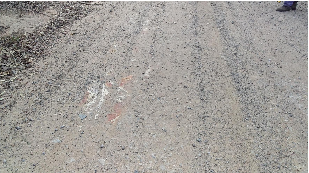
Section 1 Lot 5, Local gravel with Bitumen emulsion. Has not been reworked, good condition, no anticipated maintenance for at least 4-6 months.
