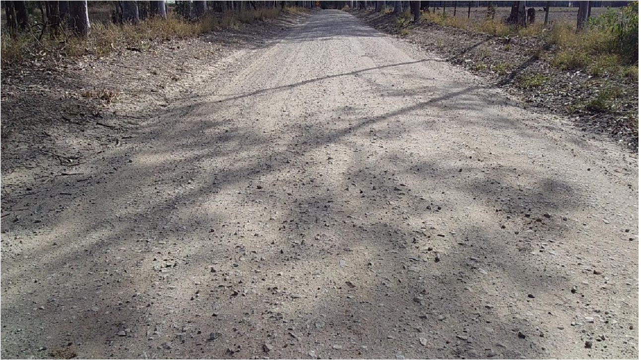
Section 1 Lot 5, Local gravel with Bitumen emulsion. Has not been reworked, good condition, no anticipated maintenance for at least 4-6 months.
