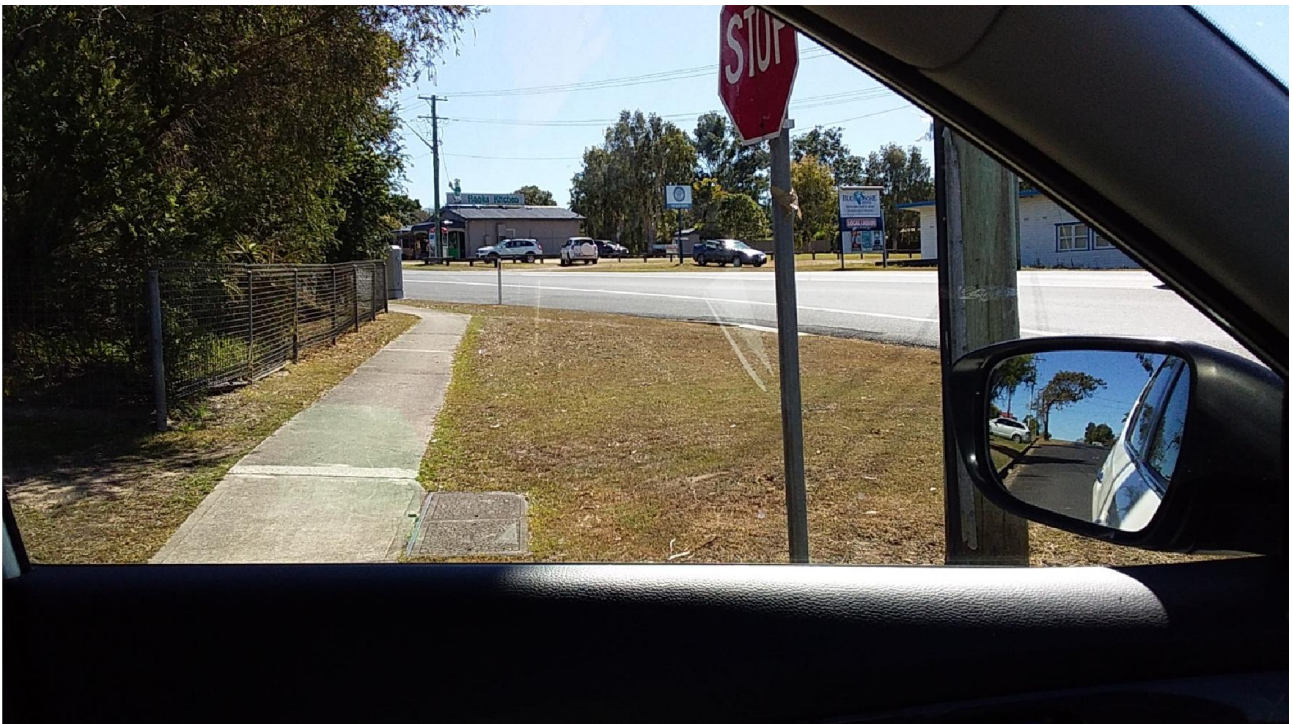
Looking left from Pine St back up The Summerland Way. If vehicles are parked legally in this location there is no sight distance to vehicles coming down the hill from the left.
