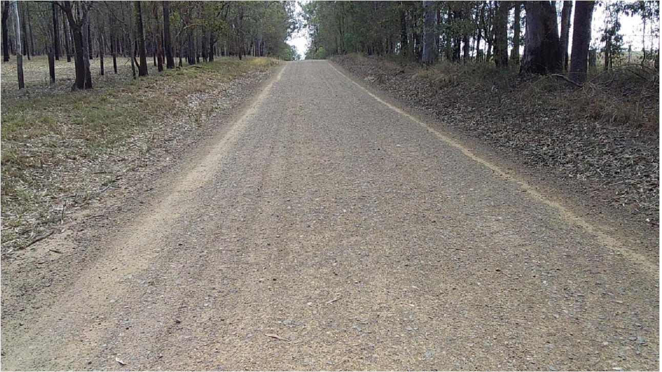
Section 2 Lot 2 – Imported Gravel to specification. Excellent shape, no defects, minimal loss of small stone and fines. No work proposed with 4 -6 months at least. That will be at least 18 months.
