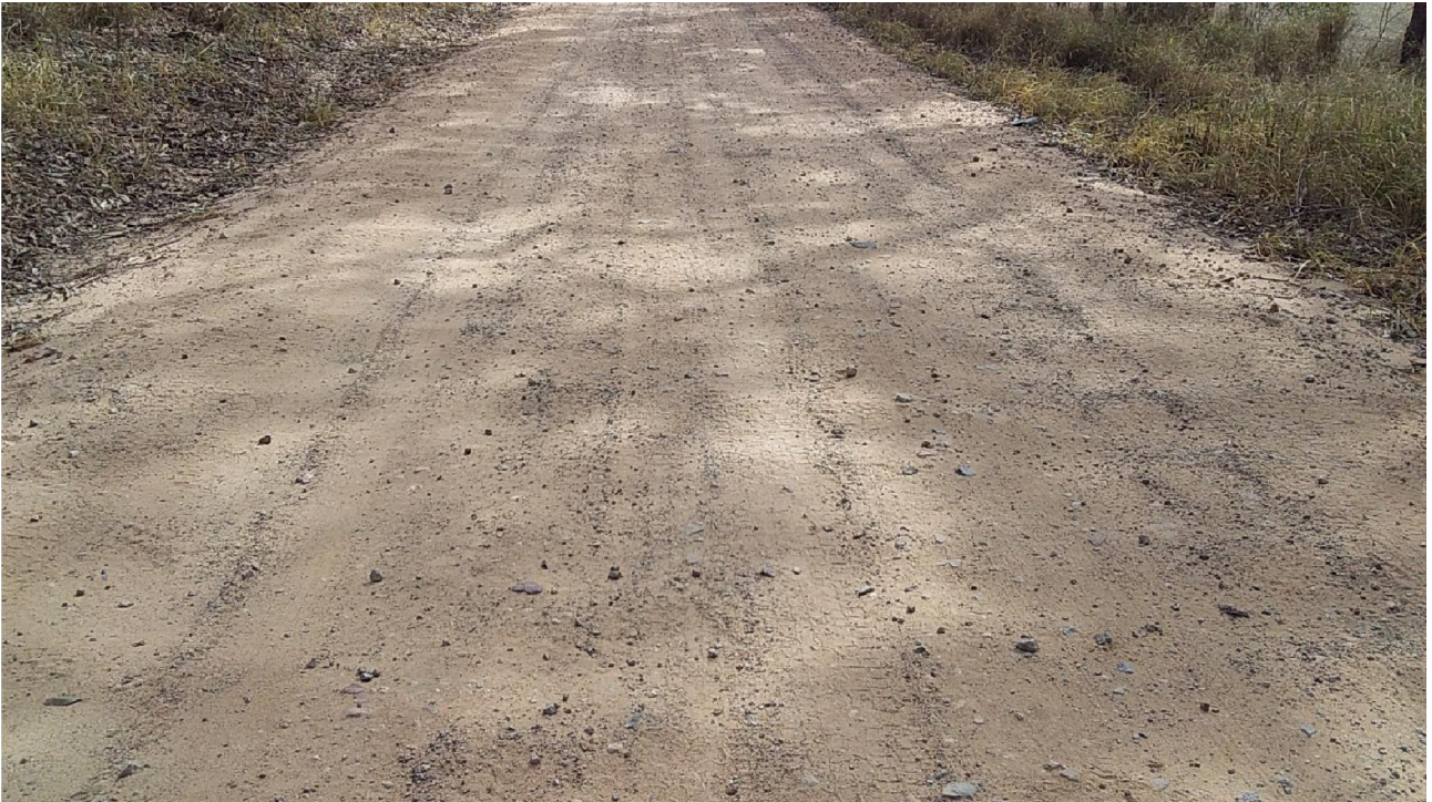
Section 2 Lot 2 – Imported Gravel to specification. Excellent shape, no defects, minimal loss of small stone and fines. No work proposed with 4 -6 months at least. That will be at least 18 months.
