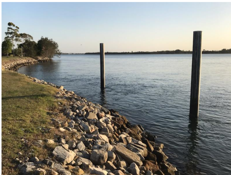
Figure 1 shows location of the existing piles looking south, the pile on the left is to be retained and made the new northern pile. (photograph by applicant)
