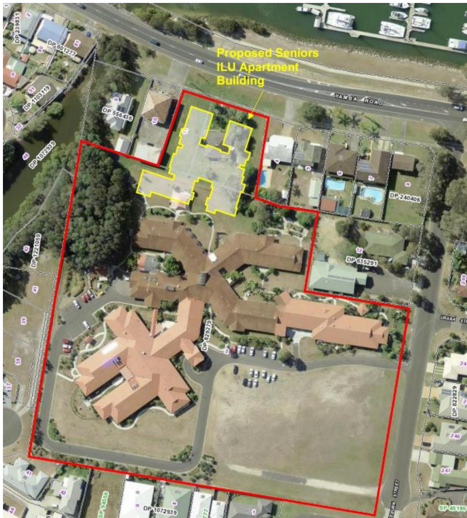
Figure 2: Aerial view of Uniting site
