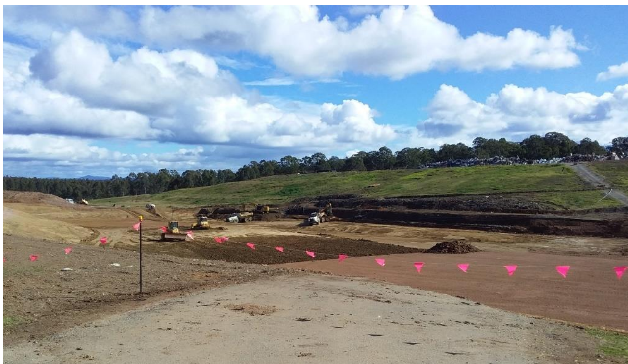
Figure 1 – Installation of clay liner
