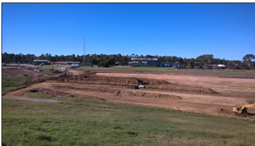
Image 1 – Bulk excavation of 180,000 tonnes clay
