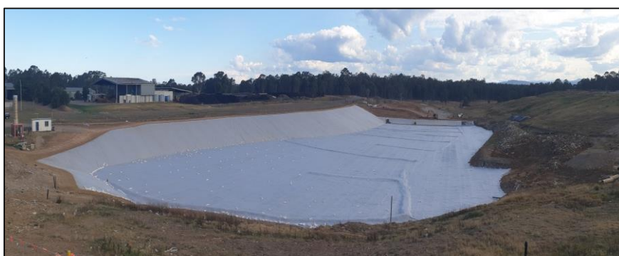
Image 4 – Installation of separation geotextile over leachate rock
