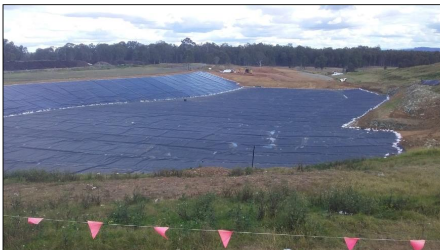
Image 2 – Installation of 2 mm HDPE Liner
