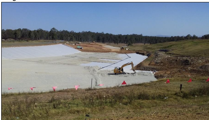
Image 3 – Installation of gravel drainage layer and leachate collection pipework over the protection geotextile
