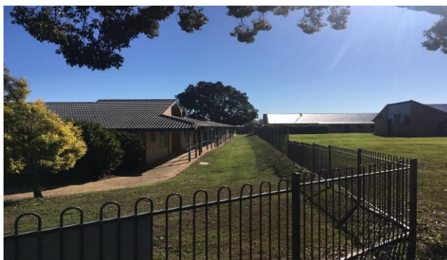
North Street frontage – Eastern boundary
