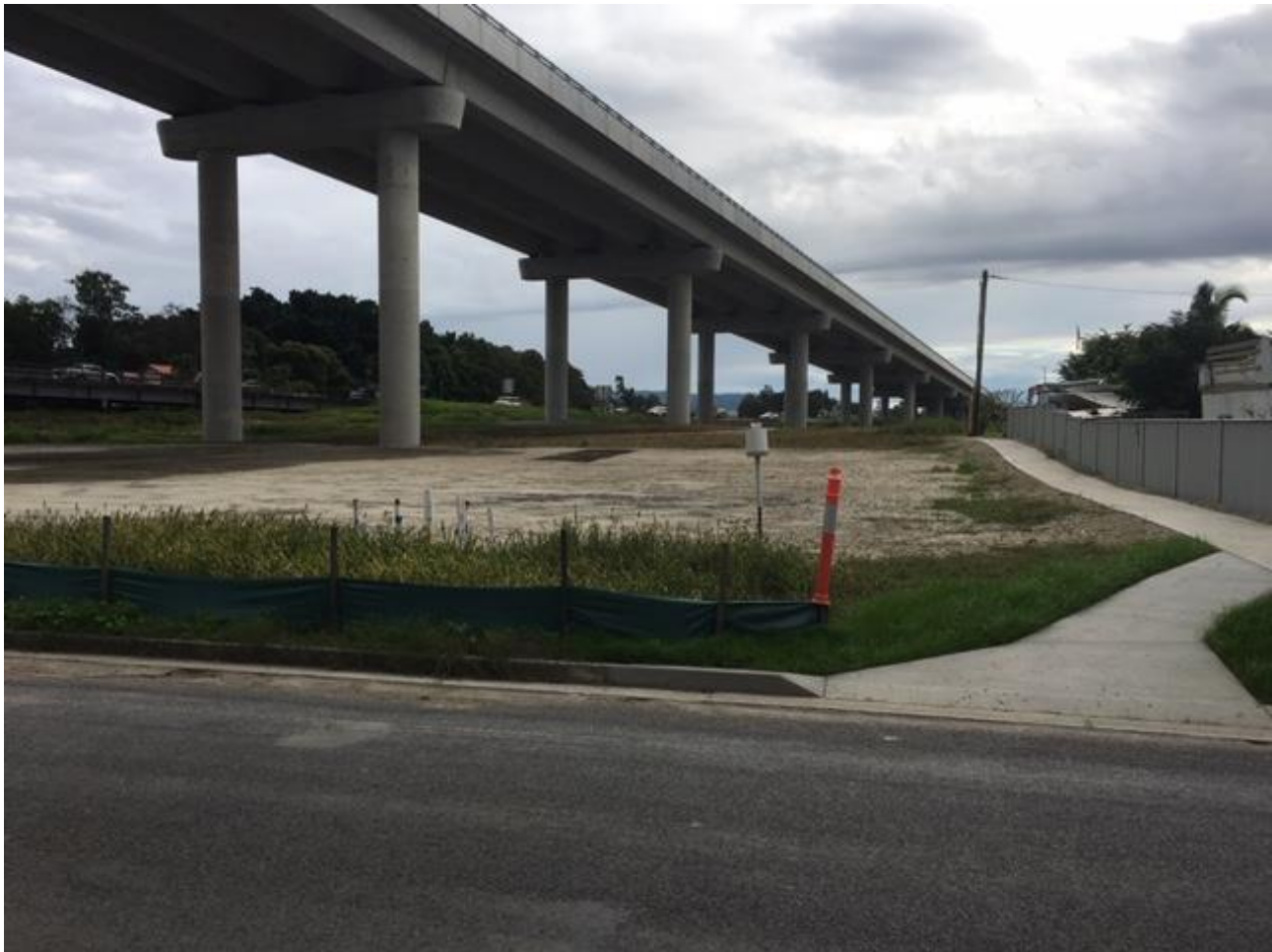
Figure 1 - Harwood Bridge Area
