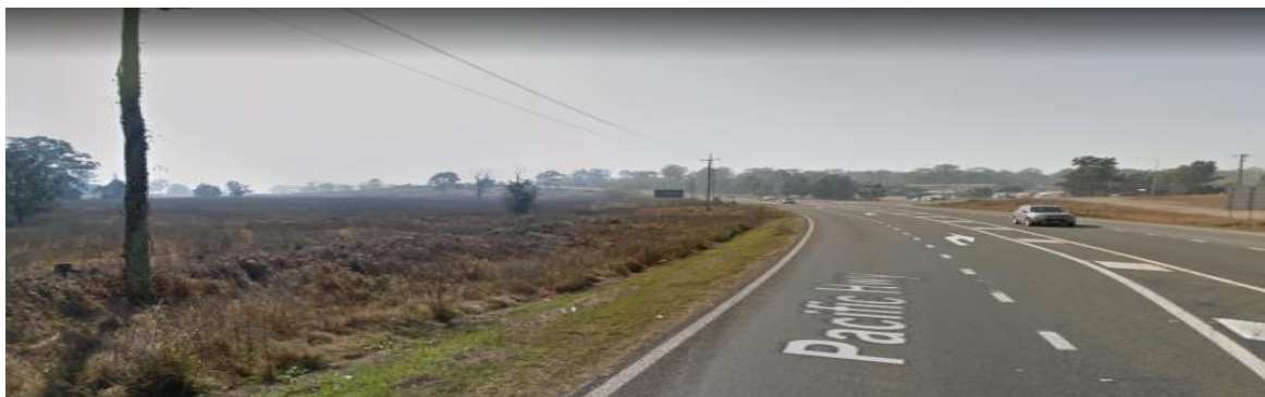
Figure 2.3 – Overhead electrical wires
