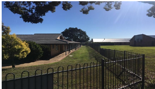
North Street frontage – Eastern boundary
