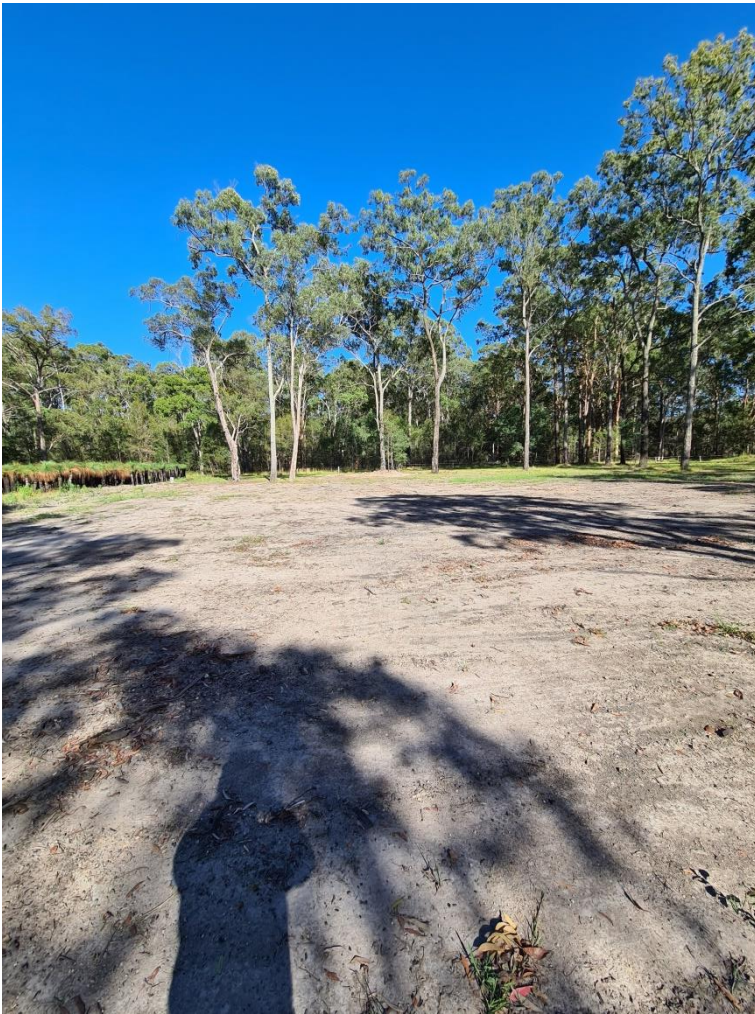
Photograph taken from eastern side of cleared area looking west across building site
