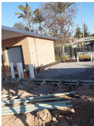
Image 2 Formwork for main slab
