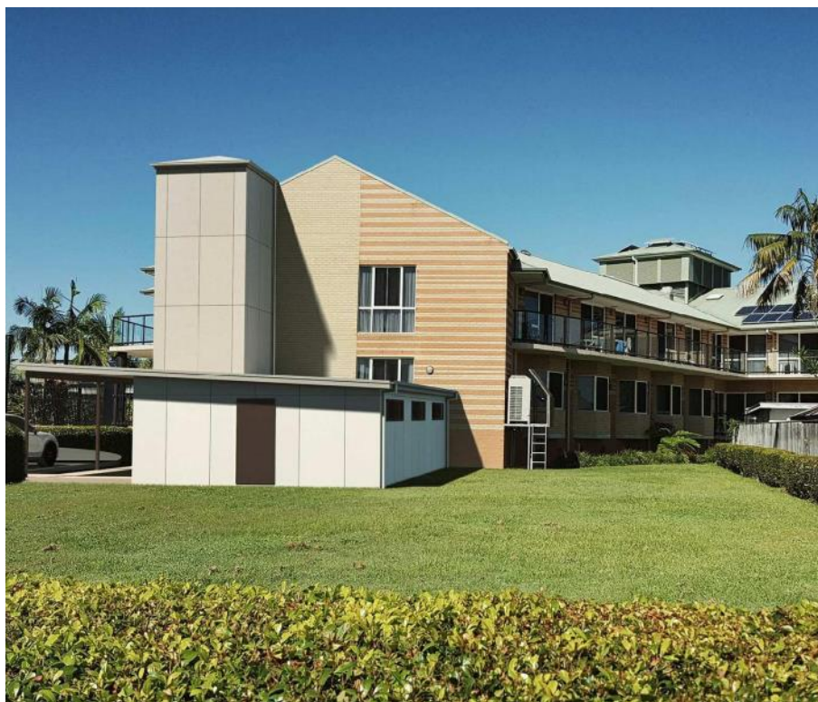
Extract of Plan by Thomson Adsett Architects Titled Perspective Lift 2 (Revision 1 dated 21 October 2019 Project No. 17.0003)
