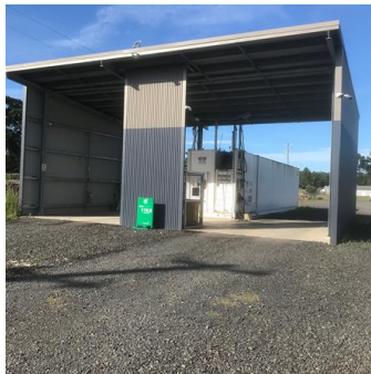
Constructed Fuel Depot
