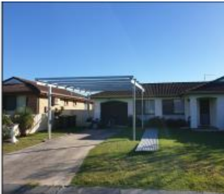
As built carport
