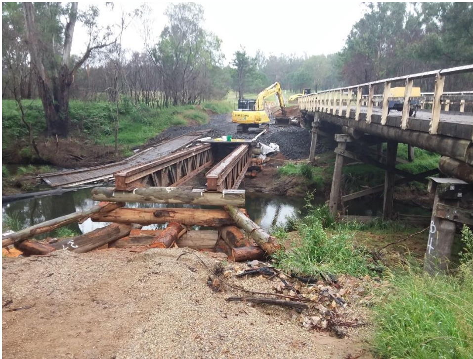
Figure 3 - Clouds Creek temporary bridge being reinstalled
