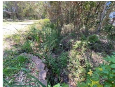
Open drain between internal road and Deering Street.
