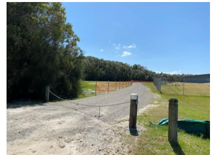
Rugby League multi-use facility gravel access Road
