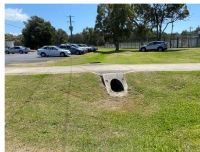
Grassed swales with concrete culvert
