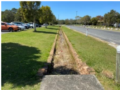
Concrete block lined drain
