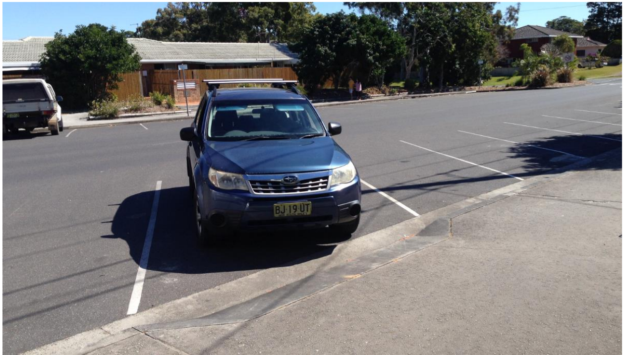
Existing layback at proposed ambulance parking bay
