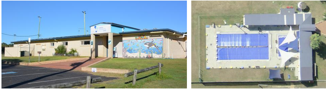
Figure 4.5: Yamba Community Heated Pool
