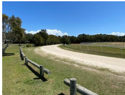
Gravel internal access road
