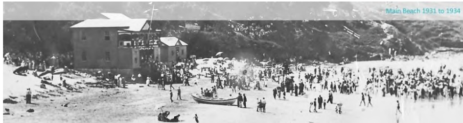
Surf lifesaving clubhouse constructed 1931 (circa 1932-1934)
