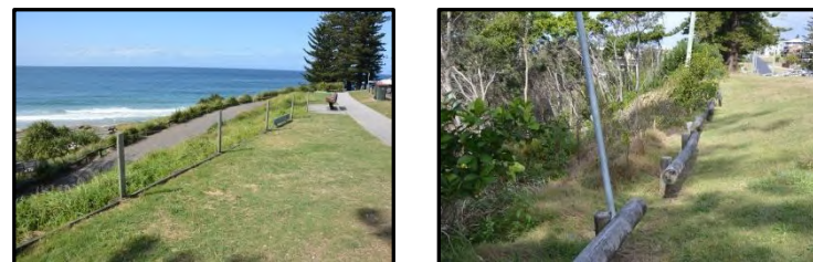
Fencing above Main Beach
