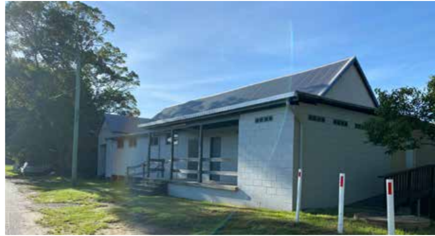
Historic Harwood Water Brigade Hall (1906) is used for well used for weddings, funerals, school activities (Harwood and Chatsworth schools), line dancing, ballet, ANZAC day ceremonies, farmers meetings. It's elevated position means it has never flooded.
