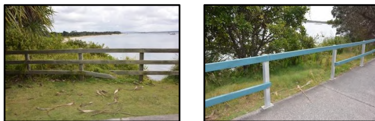
Fencing Wooli Park/Turners Beach
