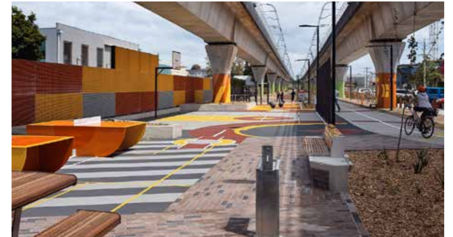
Underbridge playspace (Caulfield to Dandenong ASPECT Studios)
