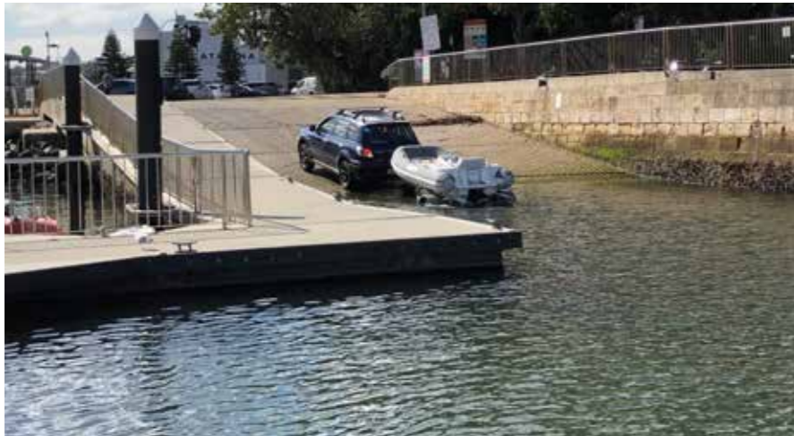
New boat ramp and pontoon (Rose Bay)
