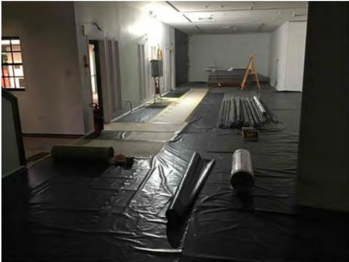
Figure 8-1: Demolition works continue inside existing Gallery (5 March)
