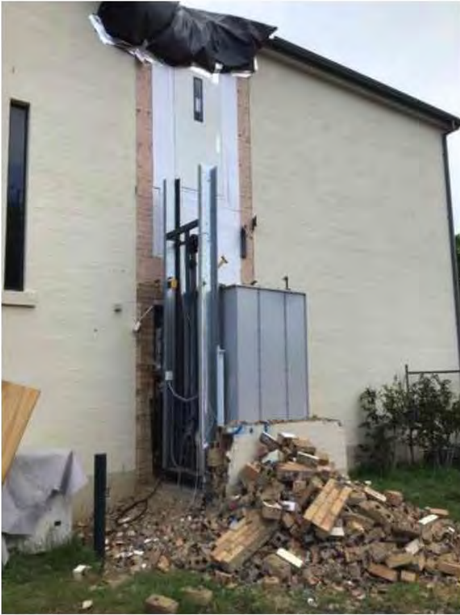
Figure 8-3: Demolition of existing Gallery lift (17 March)
