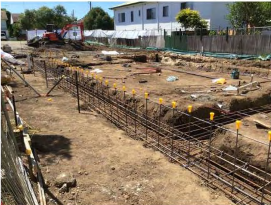
Figure 8-4: Footing reinforcement for Main Gallery extension (19 March)
