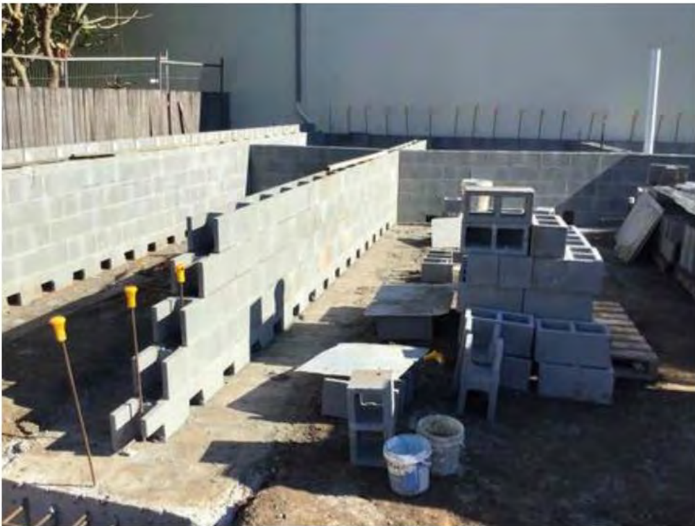
Figure 8-6: Subfloor walls for Main Gallery extension (31 March)
