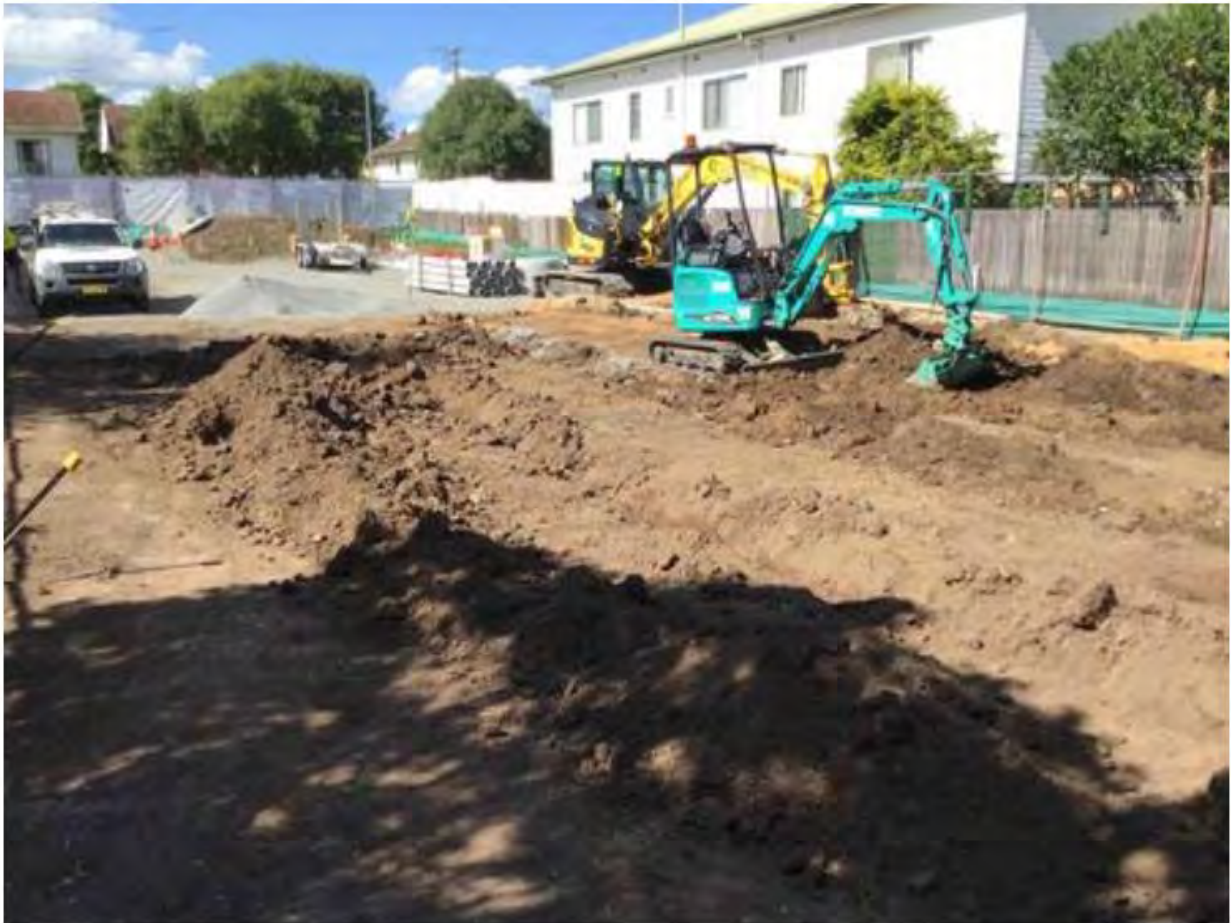
Figure 8-2: Detailed excavation for Main Gallery extension (11 March)
