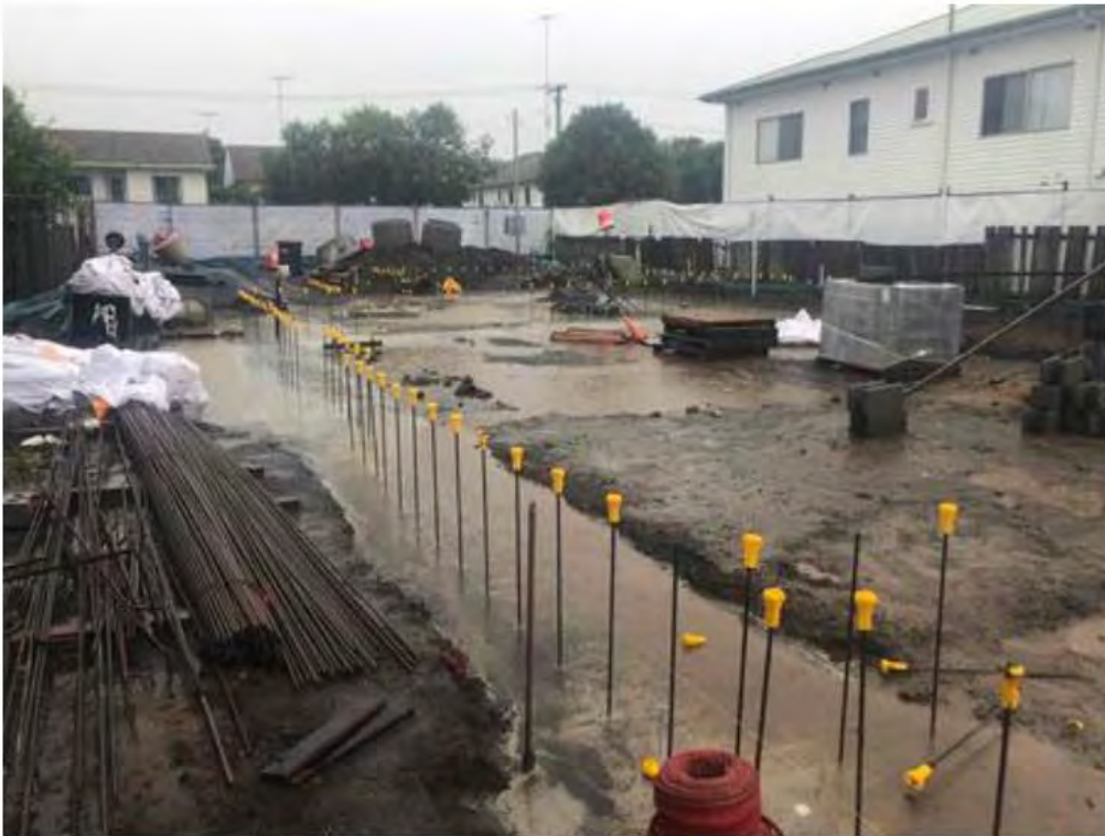
Figure 8-5: Footings poured for Main Gallery extension (26 March)
