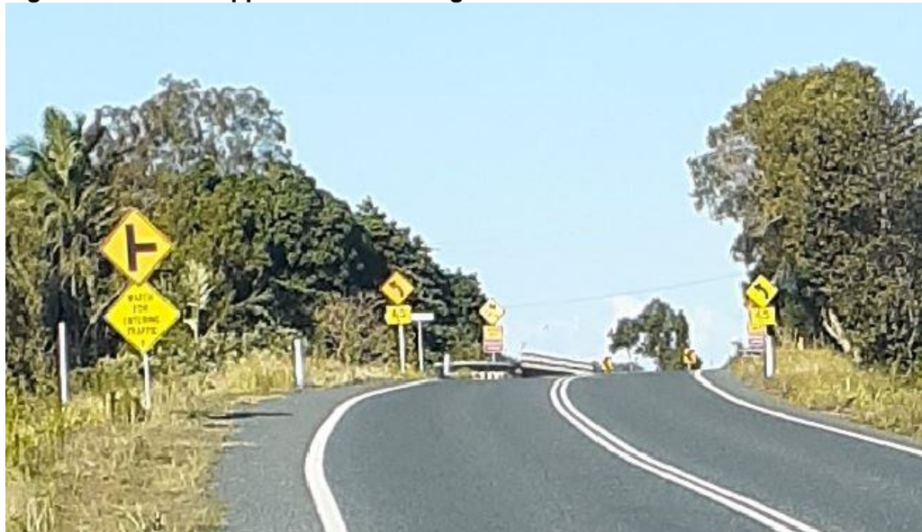
Figure 2 - View on approach to the bridge
