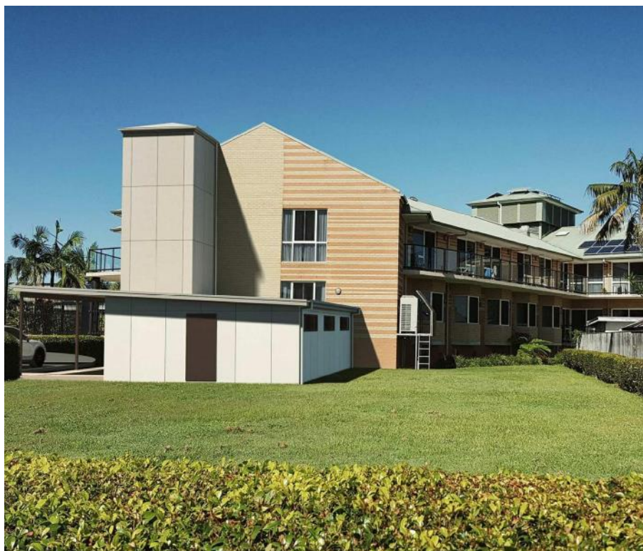
Figure 1 - Extract of Plan by Thomson Adsett Architects Titled Perspective Lift 2 (Revision 1 dated 21 October 2019 Project No. 17.003)
