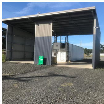
Constructed Fuel Depot
