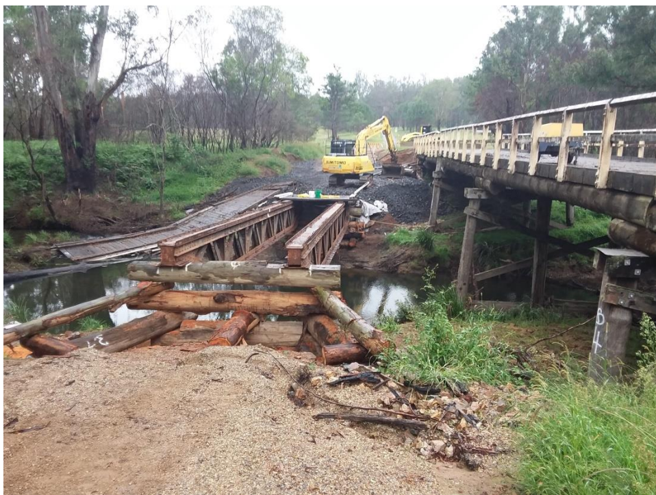
Figure 3 - Clouds Creek temporary bridge being reinstalled
