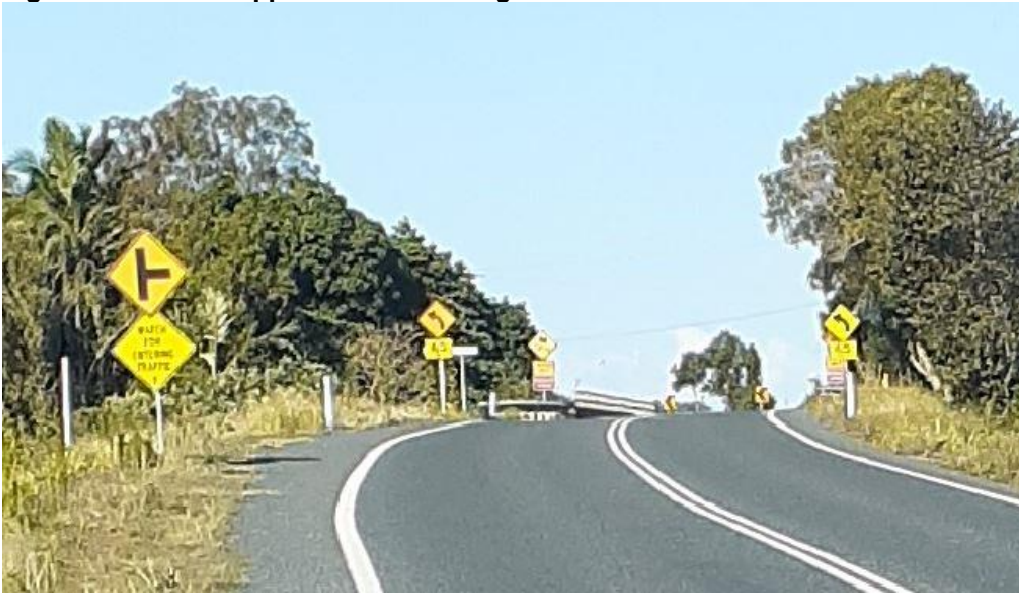
Figure 3 - View on approach to the bridge
