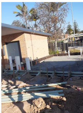
Image 2 Formwork for main slab
