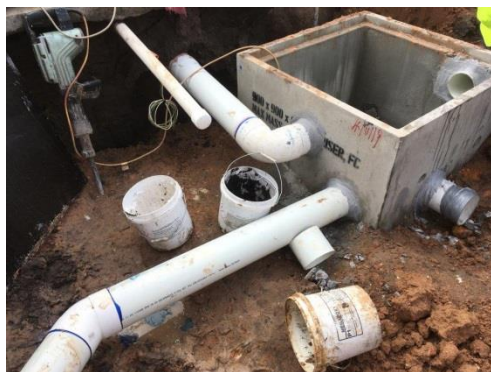
Image 1 – New pit to Pool Concourse toilet and store
