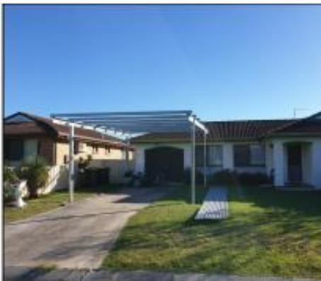
As built carport
