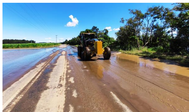
Figure 10: Council grader conducting sediment clearing on Yamba Road
