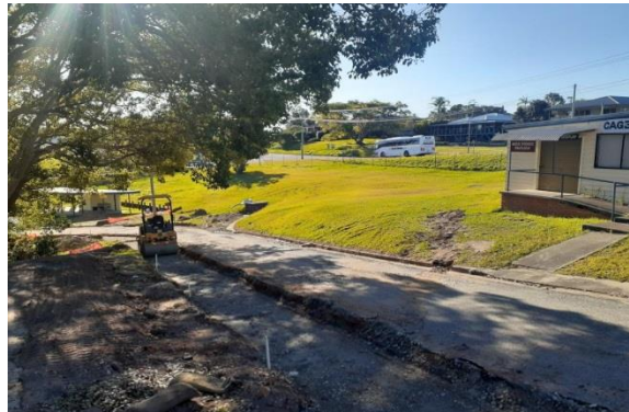
Item: Road - upgrade Location: Progress - Dump point to Main Pavilion
