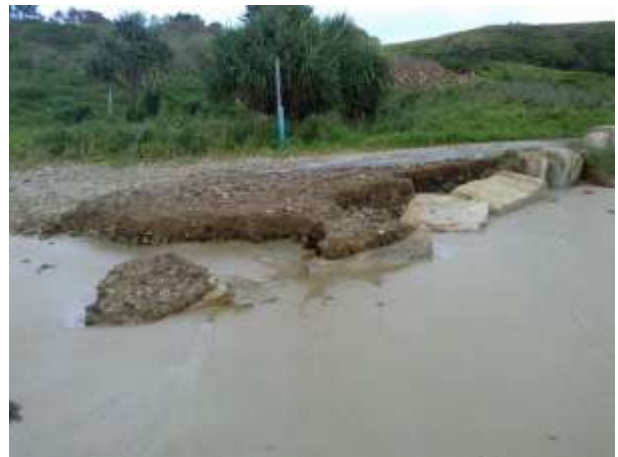
Plate 8: Localised erosion at Minnie Water beach access beside surf club (left) and boat ramp (right) - 2013
