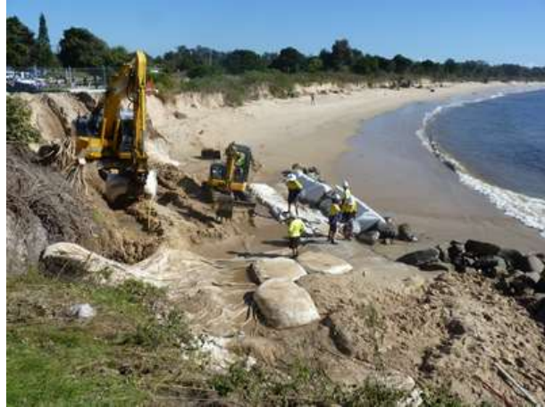
2 - Construction of GSC revetment
