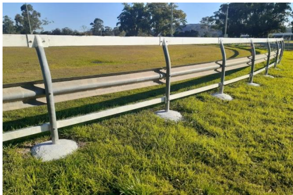
Item: Fence - repair and replacement works Location: After – Grandstand area (outside)
