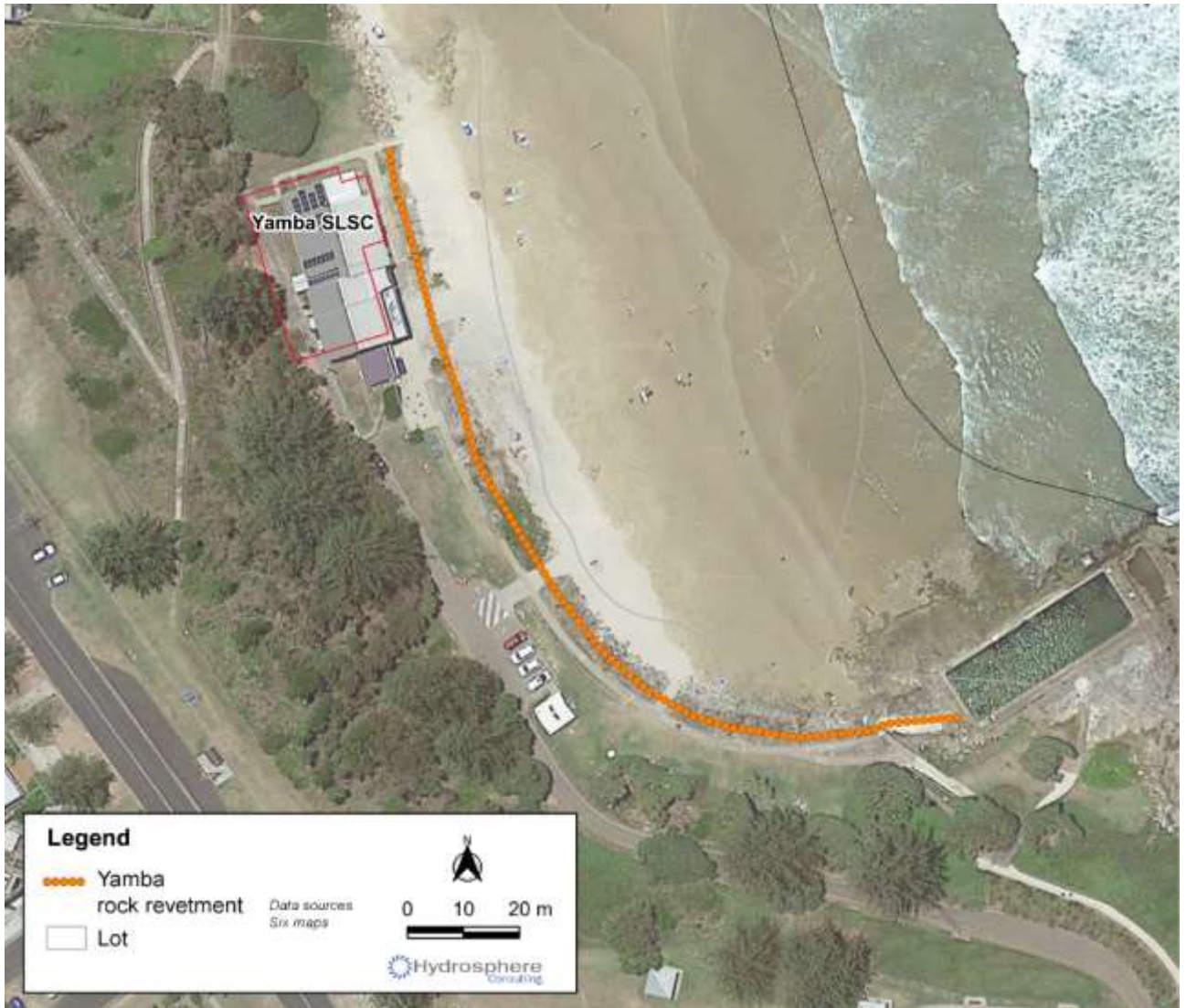
Figure 42: Location of rock revetment at Yamba Main Beach
