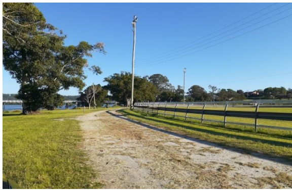
Item: Fence - repair and replacement works Location: Before – Riverfront area (outside)
