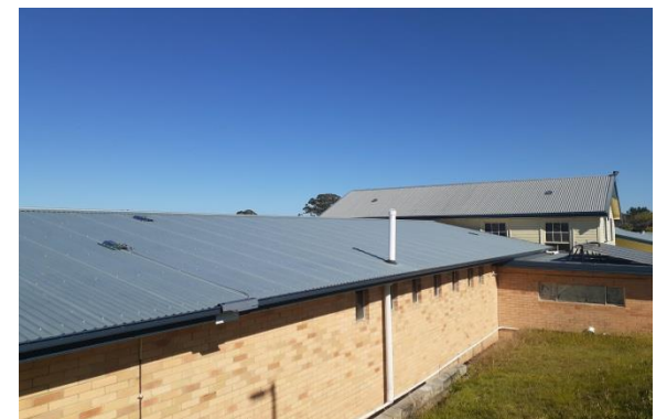
Item: Roof Access - installation Location: After – Office, Amenities, Fine Arts Building
