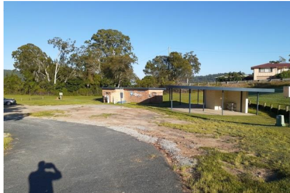
Item: Road - upgrade Location: Before - Dump point turn around
