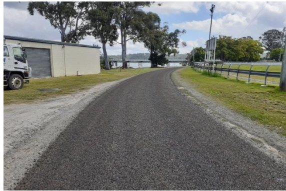
Item: Road - upgrade Location: After - Clydesdale Building to existing road
