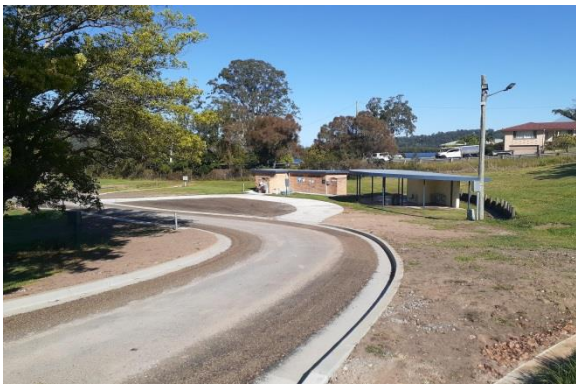
Item: Road - upgrade Location: After - Dump point turn around
