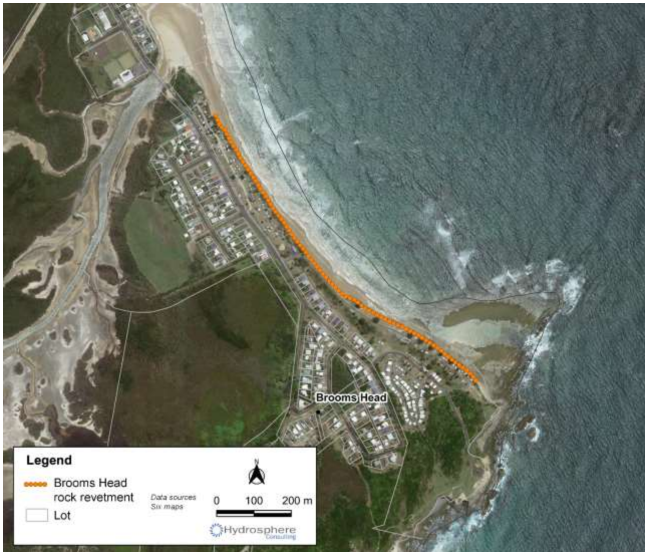
Figure 43: Current extent of foreshore rock revetment at Brooms Head
