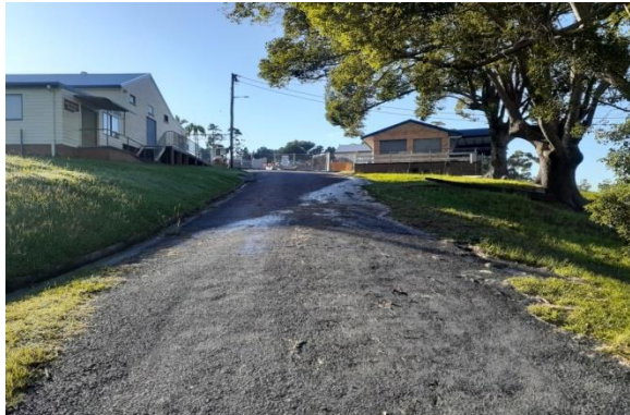
Item: Road - upgrade Location: Before - Dump point to Main Pavilion
