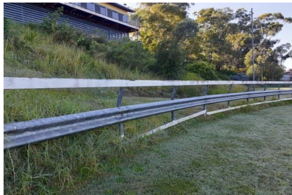
Item: Fence - repair and replacement works Location: Before – Grandstand area (inside)
