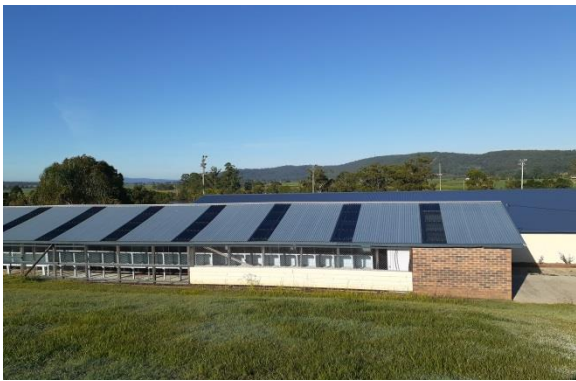
Item: Roof Access - installation Location: Before - JT Building (behind)
