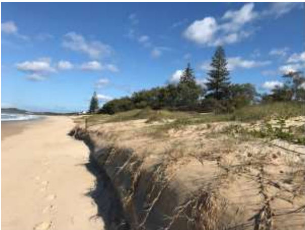
1 – Wooli Beach constructed dune
