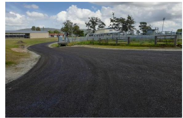
Item: Road - upgrade Location: After – Lower gate to Clydesdale Building
