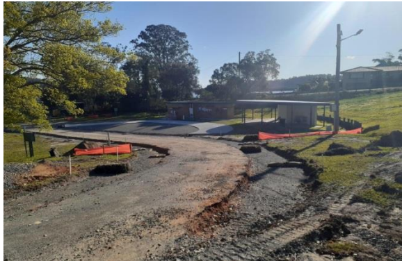
Item: Road - upgrade Location: Progress - Dump point turn around
