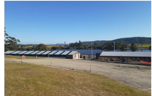
Item: Road - upgrade Location: Progress – Top car park
