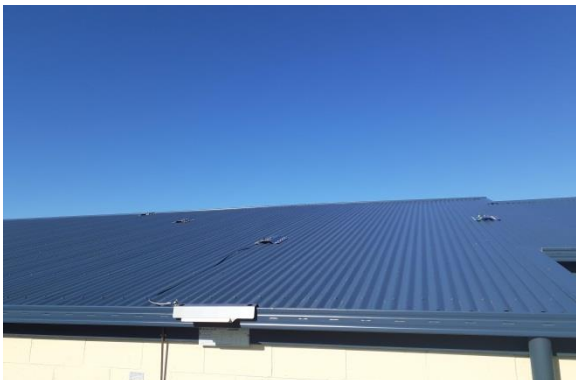
Item: Roof Access - installation Location: After - JT Building
