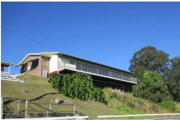
Item: JT Building - gas bottle relocate & new awning Location: Before - existing uncovered veranda
