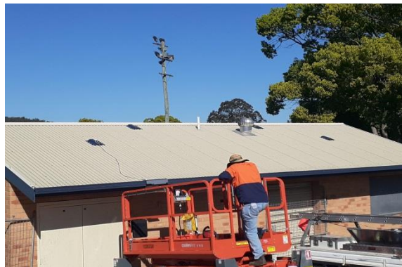
Item: Roof Access - installation Location: After - Canteen Building
