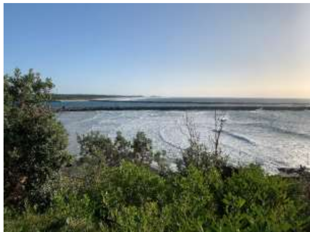
6 – Clarence River entrance breakwaters
