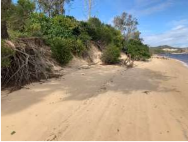
1 - erosion downstream of boat ramp
