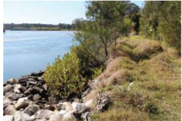
2 - Rock fillets in Romiaka Channel installed in 2008 showing good mangrove recruitment, photo from 2013
