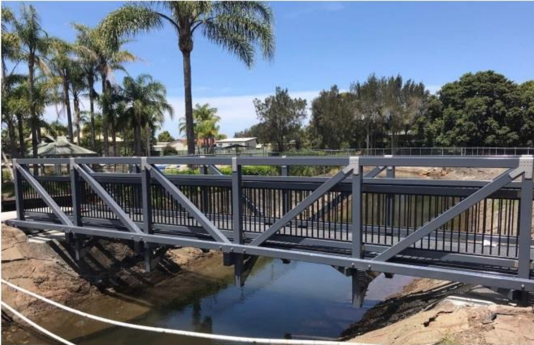
Image One – Village Resort Bridge, Port Macquarie
