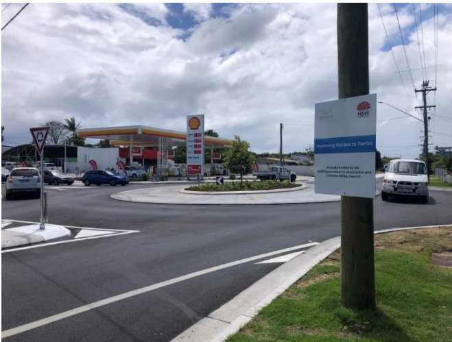
Figure 1: Treelands Drive Roundabout November 2020
