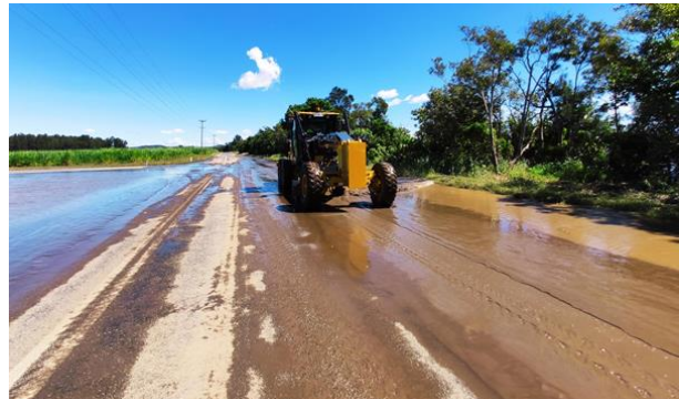
Figure 10: Council grader conducting sediment clearing on Yamba Road
