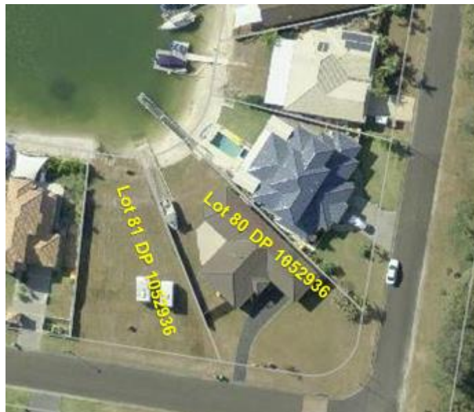
Figure 2 An aerial image of the pontoon and boat ramp at Lot 81 DP 1052936, circa 2012
