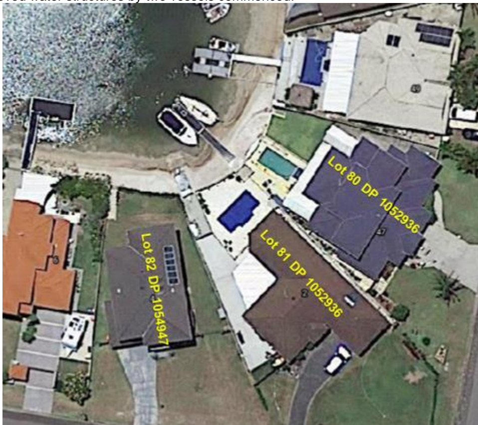
Figure 3 An aerial image of two water structures in use at Lot 81 DP 1052936, prior to construction of the pontoon at Lot 82 DP 1054947, circa 2015-2016
