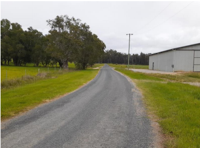
Figure 1: Existing bitumen sealed road in Bee Eater Lane, looking west from Old Murrayville Road
