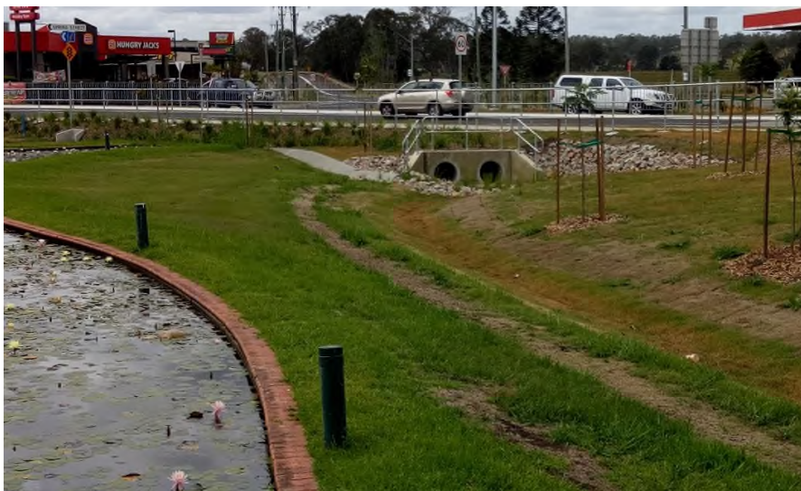
Council Stormwater Drainage
