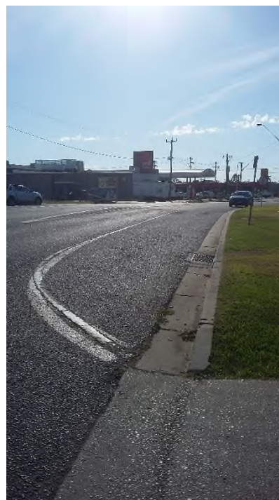
Spring Street looking east from site exit
