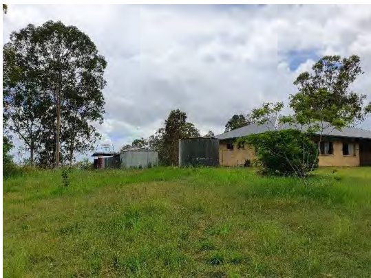
Plate 2.1 Photo looking south-east showing existing house (proposed lot 1)
