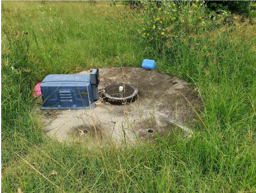
Plate 5.2 Secondary AWTS, no obvious signs of system failure/ leakage
