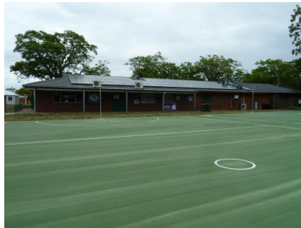
Photo 2 [rear of building]
