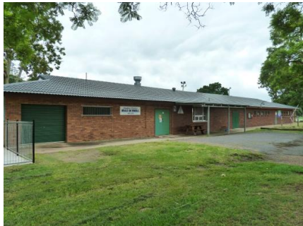
Photo 1 [front of building]
