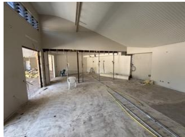
Figure 6: Electrical rough in, front of house
