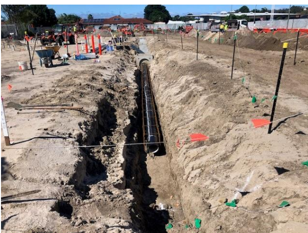
Figure 1: Stormwater pipe installation
