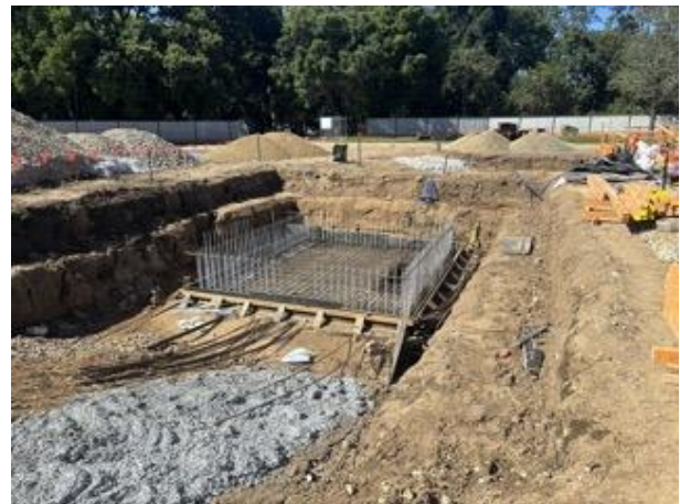
Figure 4: Steel reinforcement
