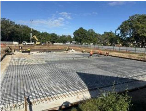
Figure 3: Steel reinforcement in the 50m pool splashpad balance tank base
