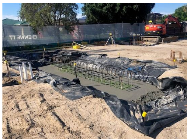
Figure 2: Concrete placed in spread footing
