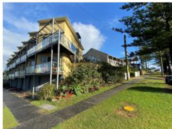
Figure 9 - Clarence Street – Looking NW
