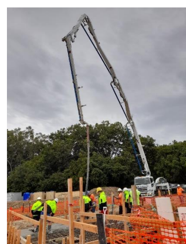
Image 7: Pouring the Splashpad lid
