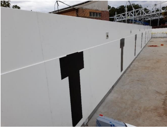
Image 1: Myrtha pool in progress – 50m pool
