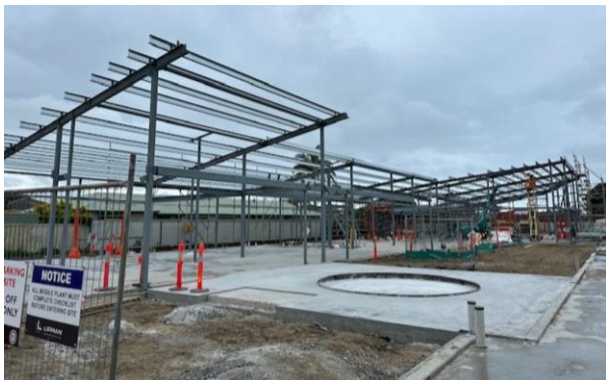
Figure 1: Steel frame, northern side of building
