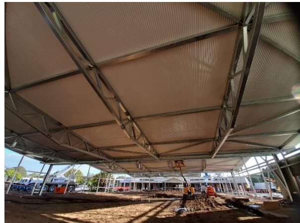
Image 4: Roof in progress, 50m pool
