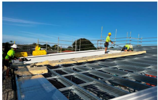
Figure 2: Roof sheeting, north-eastern part of the building
