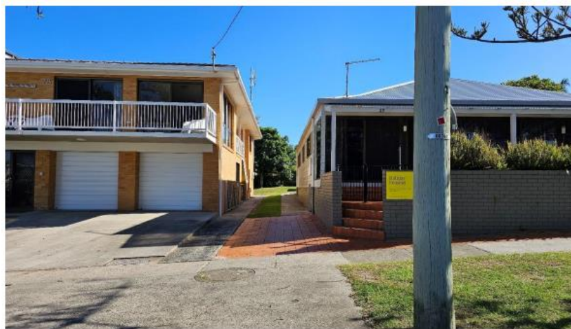
Figure 7 - 28 Clarence Street – adjoins site to the left
