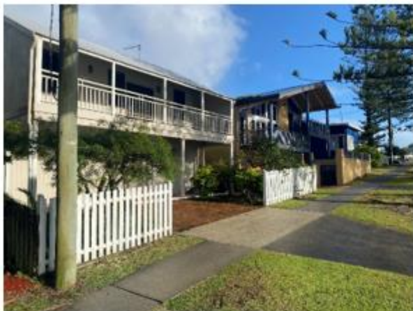
Figure 8 - Clarence Street – Looking NW
