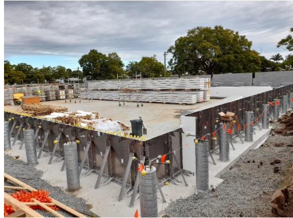
Image 2: Support structure for the Myrtha system, 50m
