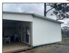
PHOTOGRAPH 3: Existing quarry office
