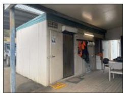
PHOTOGRAPH 5: Existing quarry lunch room
