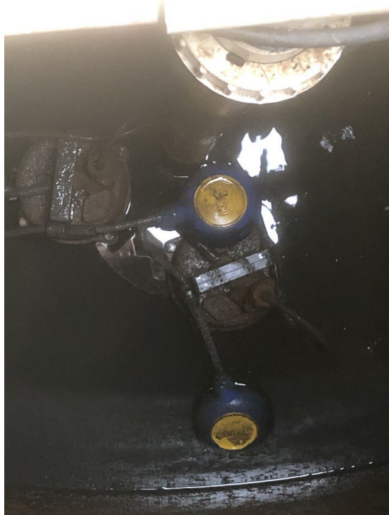
Figure 7. Float tangling due to poor design and limited tank space.
