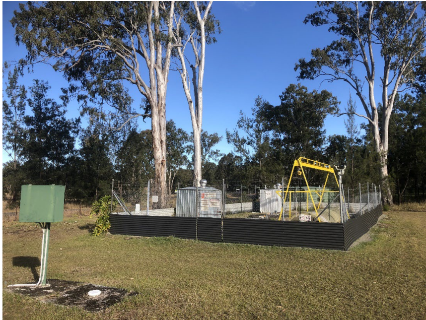
Figure 1. Baryulgil Sewage Treatment Plant.
