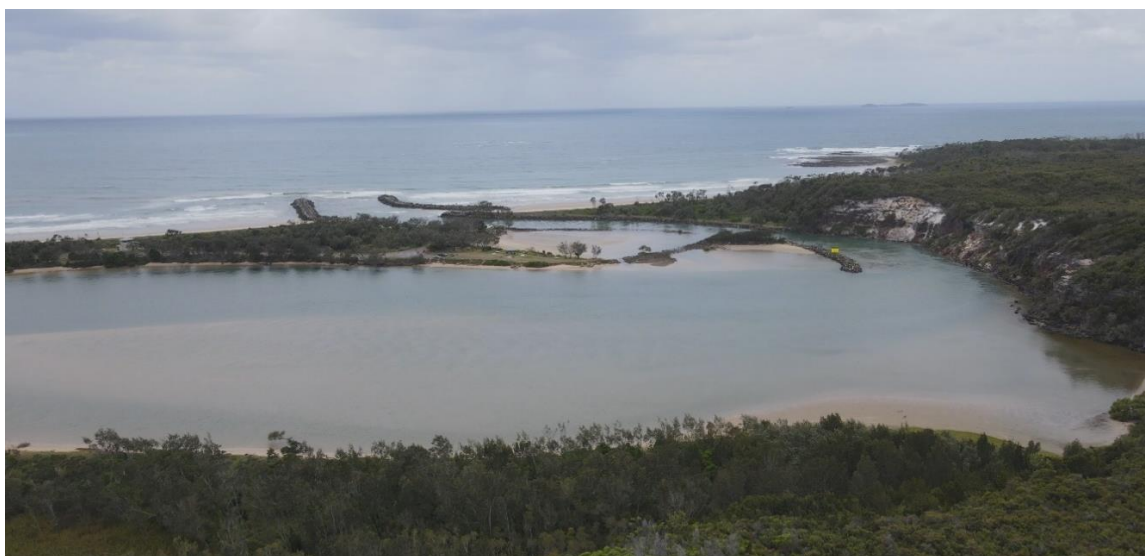
Figure 1-2: Wooli Wooli River lower estuary and training walls
